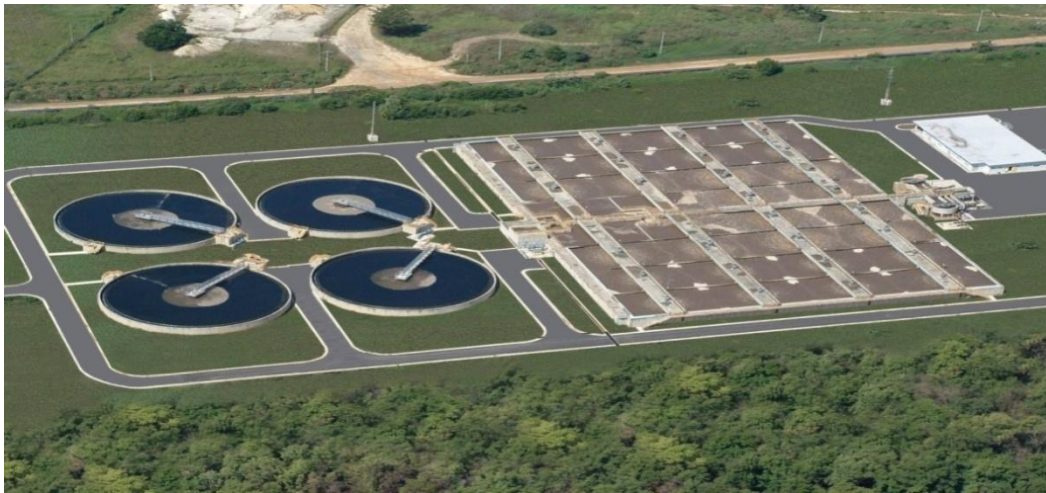
Figure 2: Aerial view of Beetham Wastewater Treatment Facility
