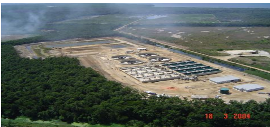
Figure 30: Newly Constructed Beetham Wastewater Facilities
