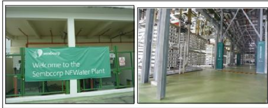
Figure 27: Changi (Sembcorp) NEWater Plant
