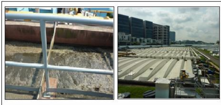
Figure 26: Ulu Panan Water Reclamation Plant in Singapore
