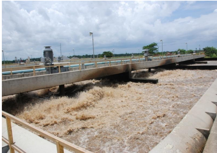
Figure 21: Typical Bioreactor
