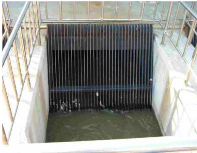
Figure 19: Typical Bar Screen
