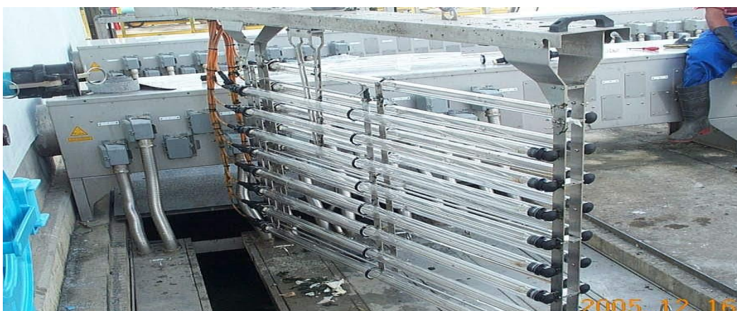
Figure 33: Low Pressure/ High intensity Lamp employed in Ultra Violet Disinfection at the Beetham Wastewater Treatment Facility
