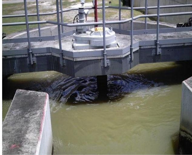
Figure 20: Typical Grit Chamber
