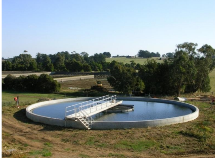
Figure 22: Typical Clarifier
