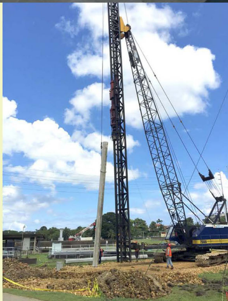
PILE DRIVING AT SITE FOR NEW SAN FERNANDO WWTP - 2015
