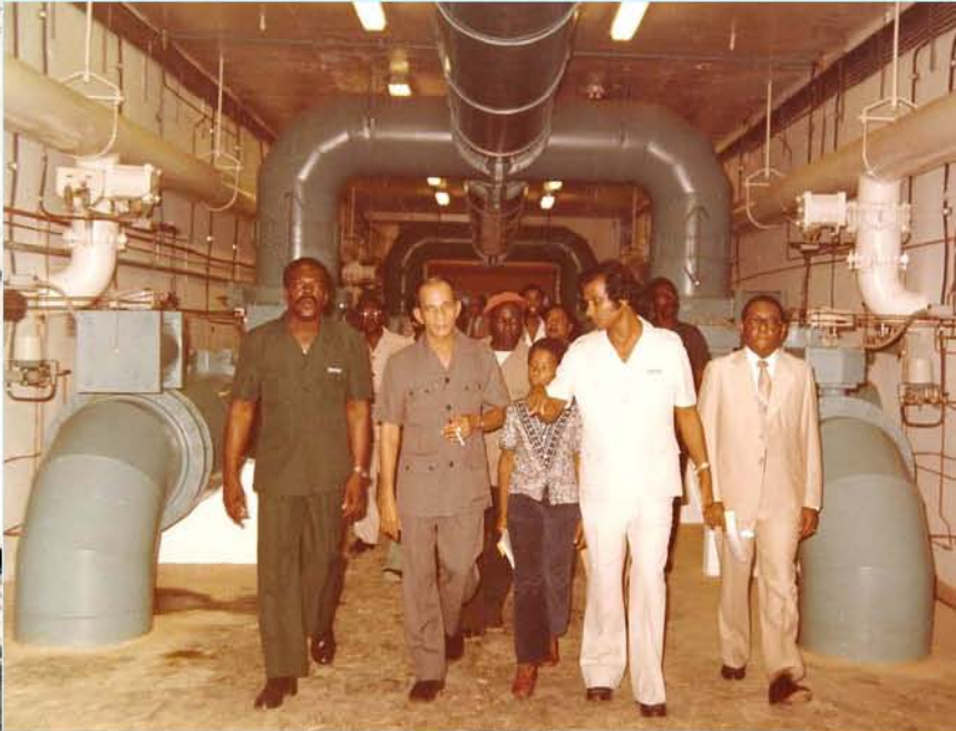
PRIME MINISTER ARTHUR NR ROBINSON AND CHIEF SECRETARY THA, NEVICK DeNOON AT COMMISSIONING OF HILLSBOROUGH WEST WTP
