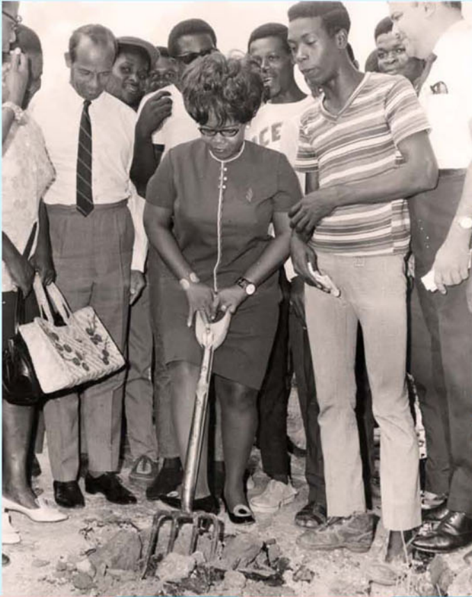
MINISTER OF PUBLIC UTILITIES MURIEL DONOWA MC DAVIDSON AT THE SOD TURNING FOR PIPELINE PROJECT
