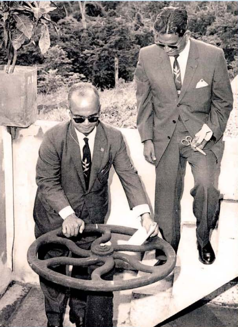
PRIME MINISTER DR. ERIC WILLIAMS AND PUBLIC UTILITIES MINISTER KAMALLADIN MOHAMMED AT COMMISSIONING OF THE UPGRADED NAVET WTP 1976
