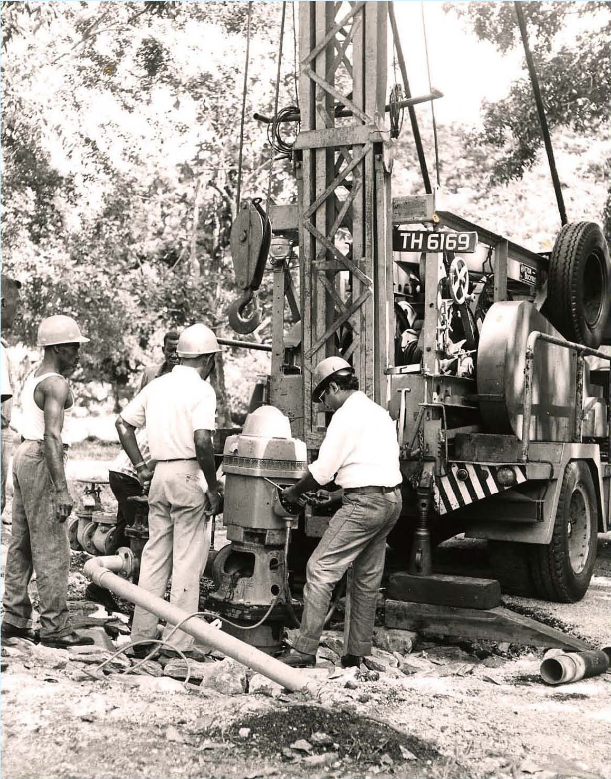
WATER WELL DRILLING 1970's
