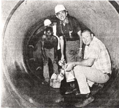
Inspecting a laid pipe.
