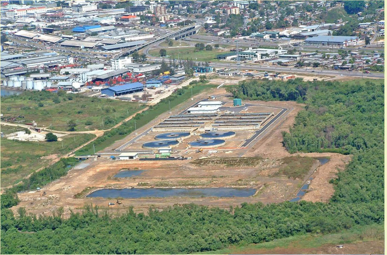
ARIEL PHOTOGRAPH OF NEW WASA BEETHAM WWTP IN 2005
