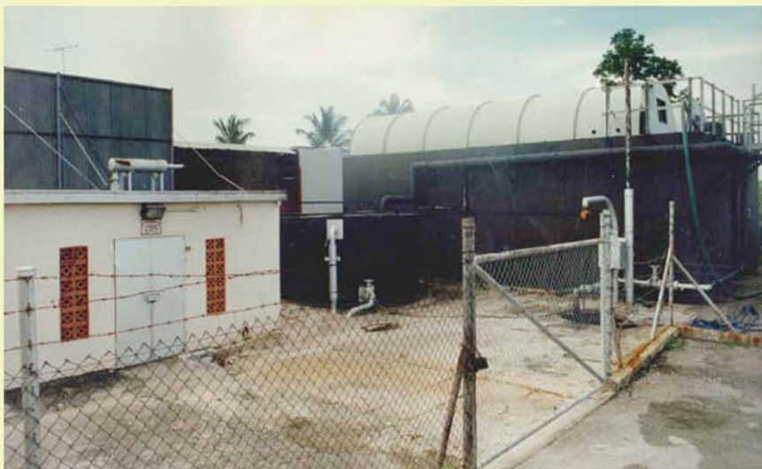
ONE OF THE HDC PACKAGED WASTE WATER TREATMENT PLANT ADOPTED BY WASA
