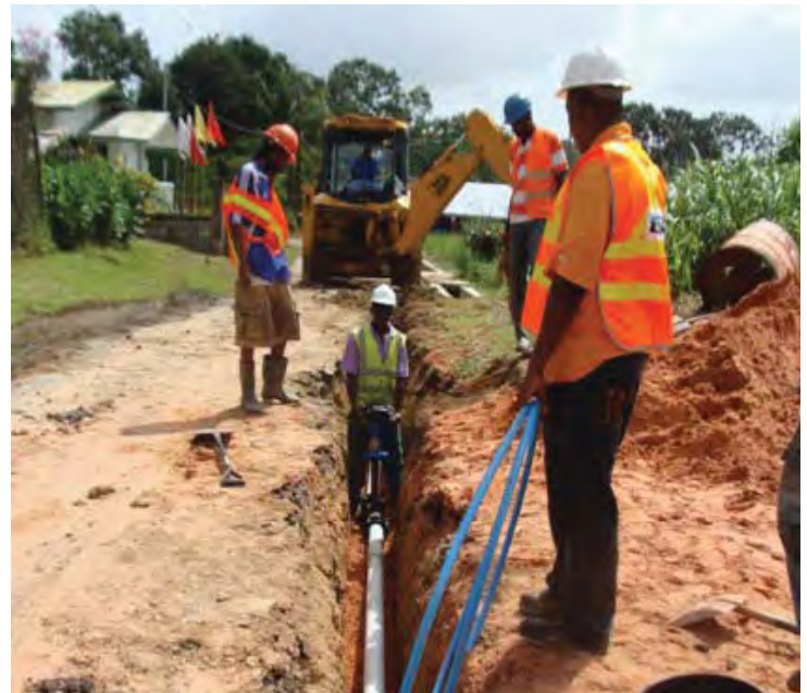
Mains Installation project in Barrackpore
