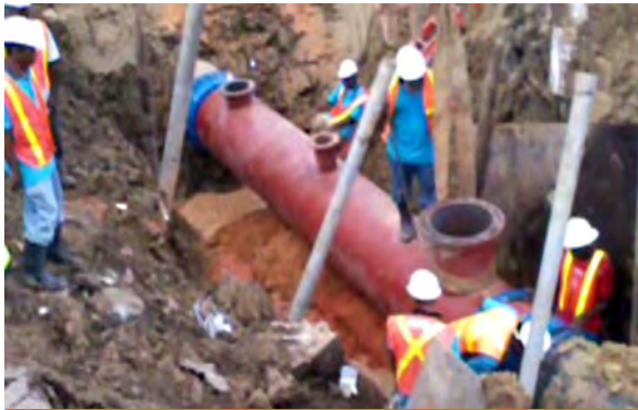
Pipeline relocation at Dumfries Junction, La Romaine
