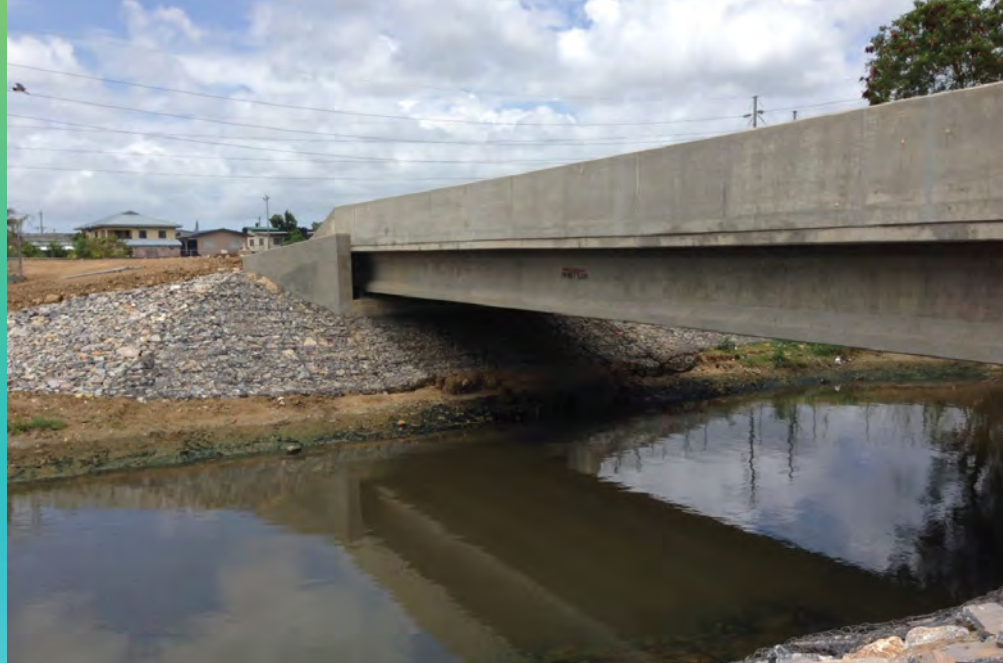
The recently completed access road and bridge to the San Fernando Wastewater Plant.
