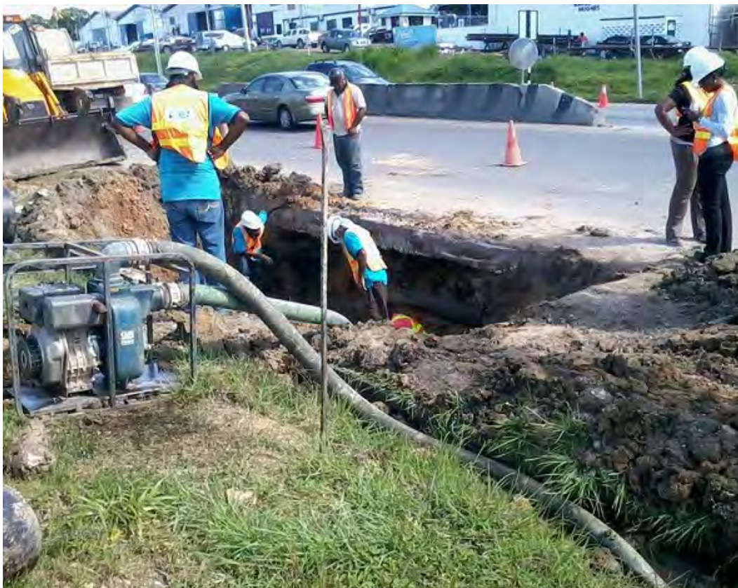
Valve installation along South Trunk Road
